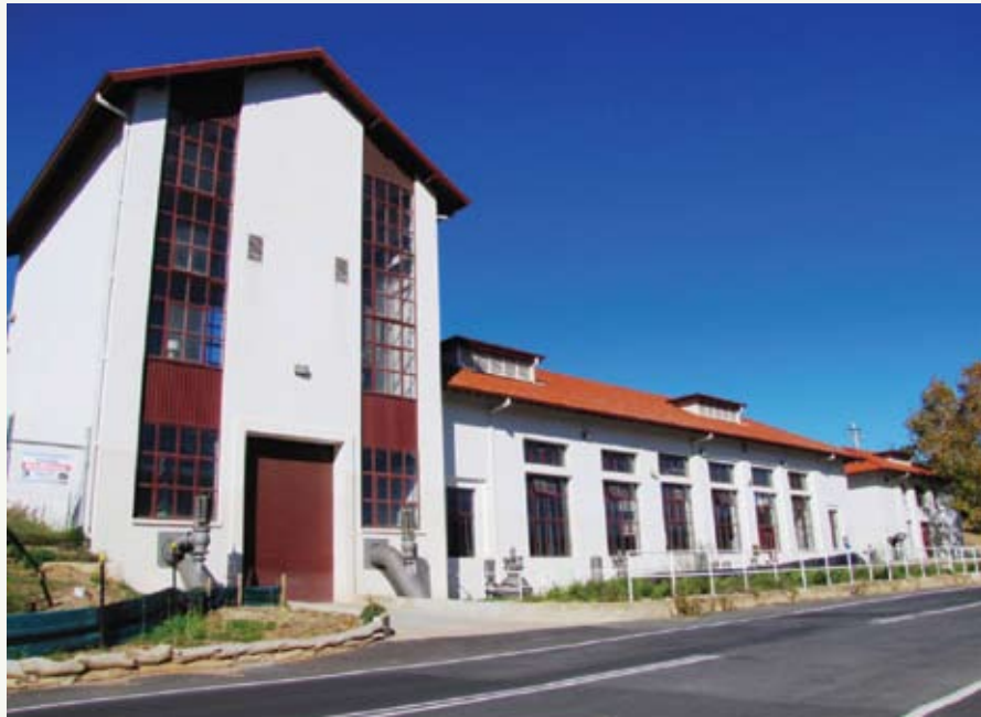
Cotter Pumping Station. Photo: Luke Johnston
