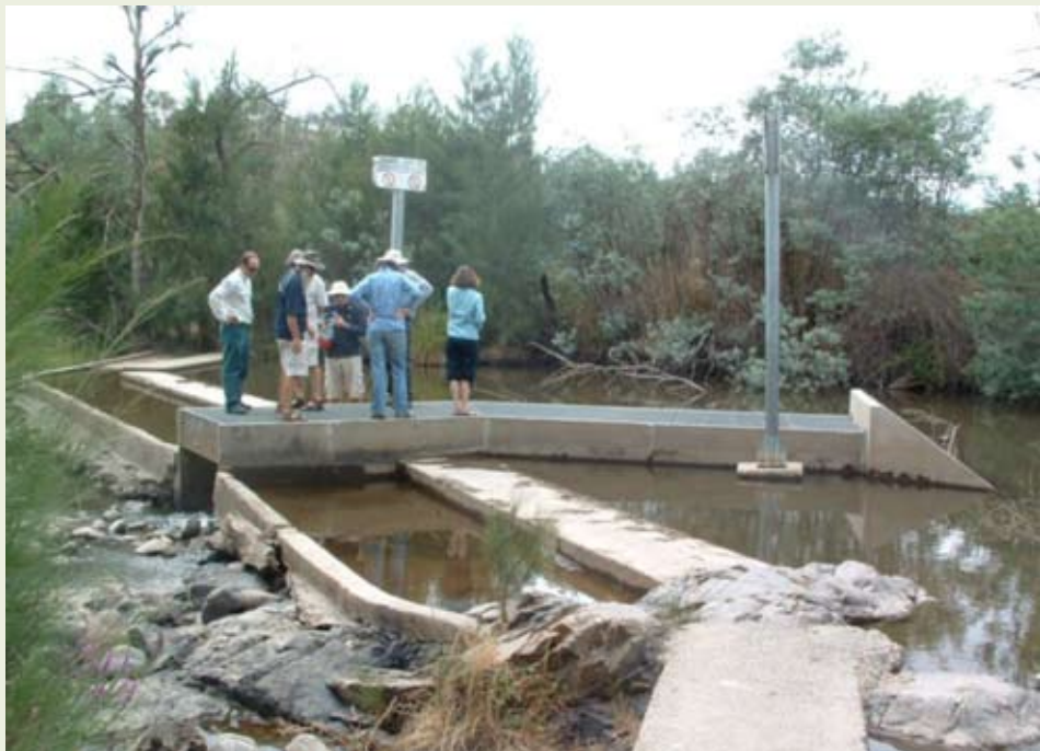
Plate 10: In-stream weir and fishway on the Cotter River near its junction with the Murrumbidgee River. Photo: Bill Phillips
