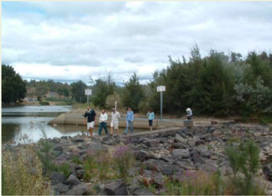
Plate 9: In-stream weir and fishway at Casuarina Sands. Photo: Bill Phillips
