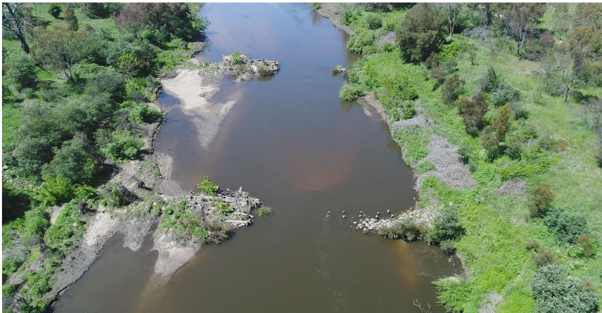
Figure 13. Previously installed engineered log jams (part of the 2011 GHD work) and an enlarged and realigned rock groyne (originally part of the early 2000s work) within the Tharwa Reach. (Photo: Hugh Allen).
