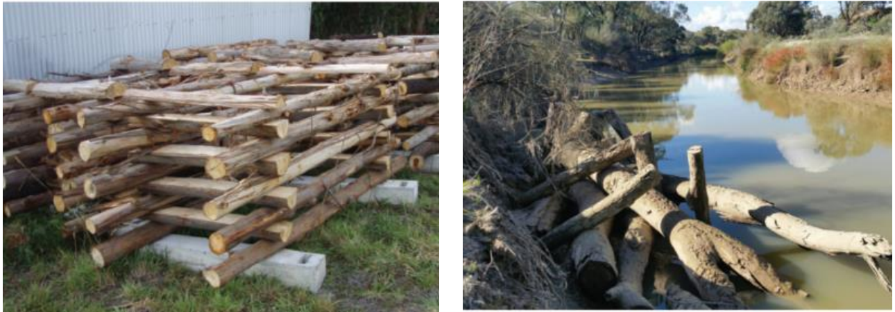
Figure 22. Types of large wood installation used for habitat improvement. (L) fish hotel, (R) large wood arrangement using two root balls and four large trunks. Source: ARI, 2019
