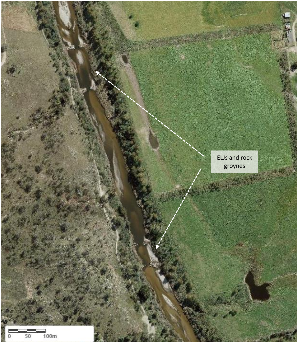
Figure 14. Aerial imagery of the Tharwa reach showing the 2013 engineered log jams, paired to enlarged rock groynes (bottom pair of structures) and the 2018 engineered log jams (top pair of structures) in February 2021 (Photo: ACT Government)
