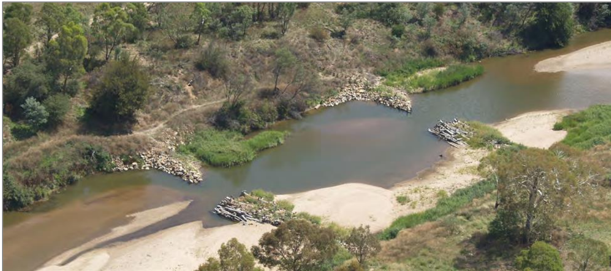
Figure 17. Aerial image of the engineered log jams at the Tharwa sand affected reach (Photo: ACT Government).
